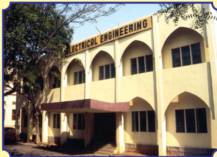
Department of Electrical Engineering
